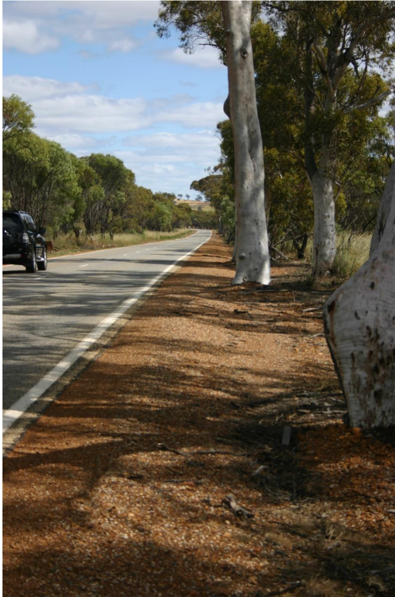
Photograph 3: Tree in foreground is 1.3m to edge of bitumen. Tree in background is 0.8m to edge of bitumen. Both trees are in excess of 50 years old.
