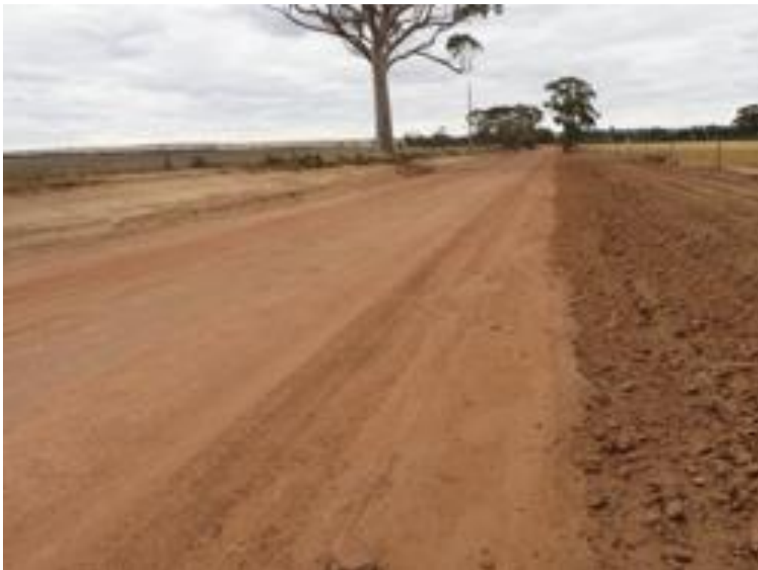
Koomberkine North Road: cleared fenceline to fenceline – for what purpose
