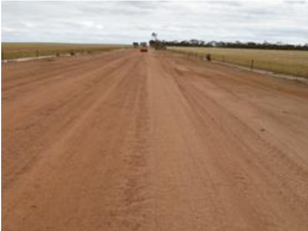
Koomberkine North Road: cleared fenceline to fenceline
