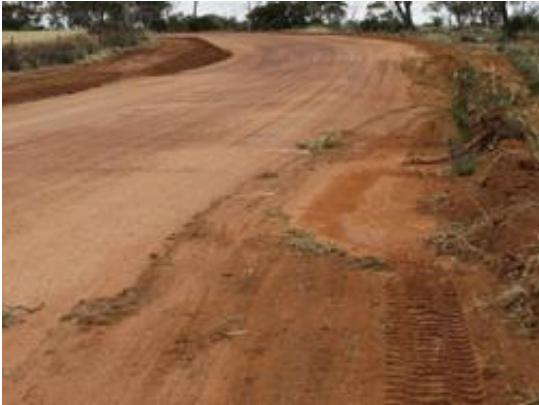
Koomberkine North Road: clearing fenceline to fenceline in areas not damaged by flooding
